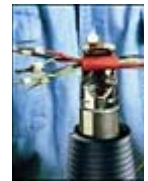
Applying Shrink Tubes
